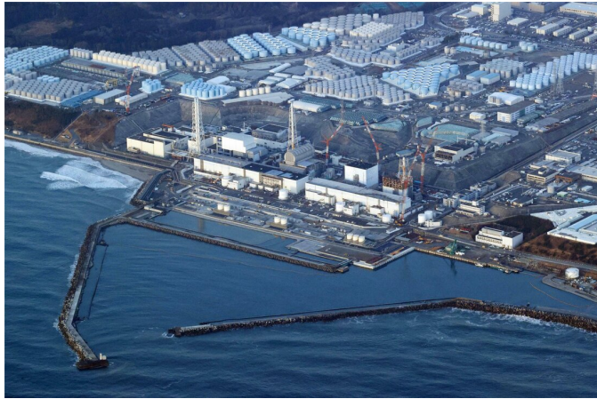
FIGURE 11. Since the Fukushima nuclear accident, over 1.3 million tons of nuclear wastewater have been collected, treated, and stored in an immense tank farm at the plant.
