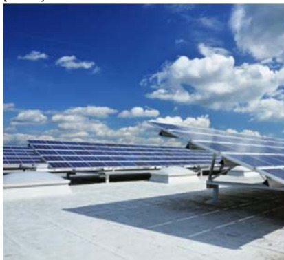
Solar Panels in a rooftop
