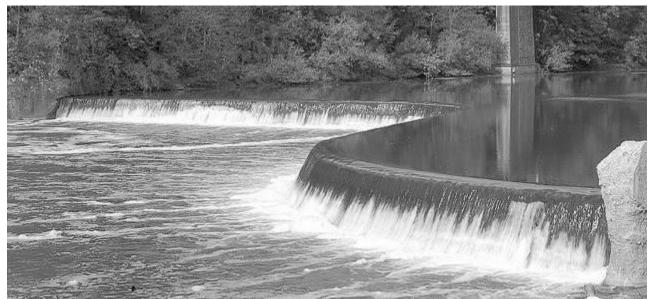
Figure 8. Curves in dams are made to increase their strength like with arches.
