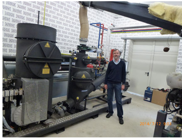
Fig. 4. Spanner Re 2 wood gas cogenerator installed by Josef Strobl Heizung Solar in Giglberg and Velden/Vils/Lower Bavaria/Germany. Left: suitable wood chips. Right: modern 100% wood to gas pyrolysis unit.
