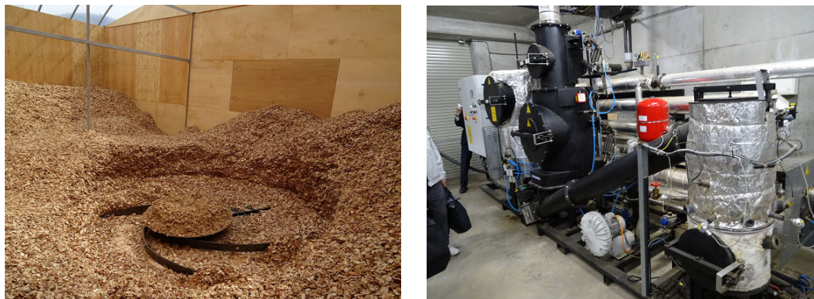
Fig. 7. Wood gas co-generator of Spanner K.K. installed 2014 in Ecomura near Koriyama, Fukushima Prefecture, Japan. Left: automatic feed-in of wood chips. Right: Spanner Re 2 pyrolysis unit (wood to gas).
