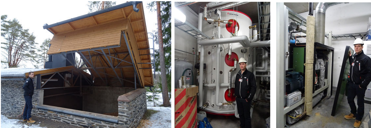
Fig. 8: Volter Oy wood gas cogenerator facilities near Kempele/Oulu/Finland. Left: hydraulic roof wood chip fuel storage. Center: warm water tank. Right: compact wood gas cogenerator. Supplying 32 residential units (see above layout drawing, blue) with total floor space of 2365 m 2 [Liikkujantie 19 2015].
