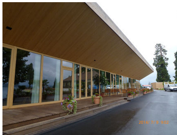
Fig. 3. Mainau Island Restaurants space heating/warm water by Wood Gas Cogeneration.
