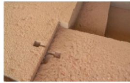
stabilizing metal pin and megaliths in the Axum (Ethiopia)
