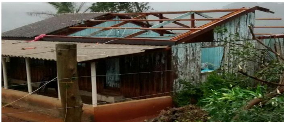
Figure-3. Photo of damage caused at home by alleged Tornado in Rosario do Ivaí [3].
