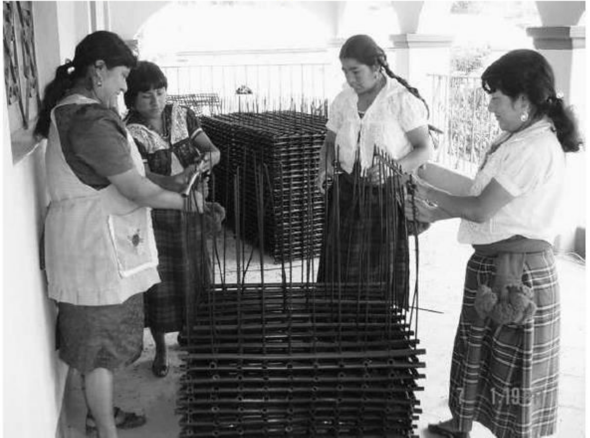
FIGURE 4 Women weaving the entrails of a community built and operated anaerobic wastewater treatment plant for recycling domestic effluents for further use for agricultural production on communal lands in a highland community in Ixtlán de Juárez, Sierra Norte, Oaxaca. (Photo courtesy of Carlos Pailles, Director, Center for Ecological Support, Huatulco, Oaxaca, Mexico)
