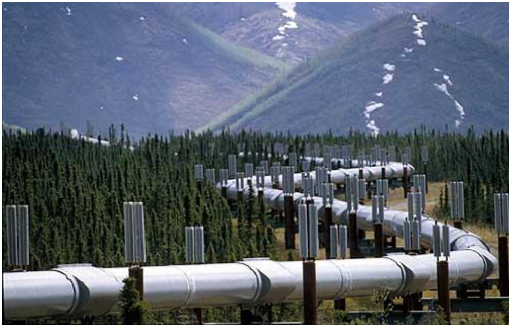
Typical ground pipeline
