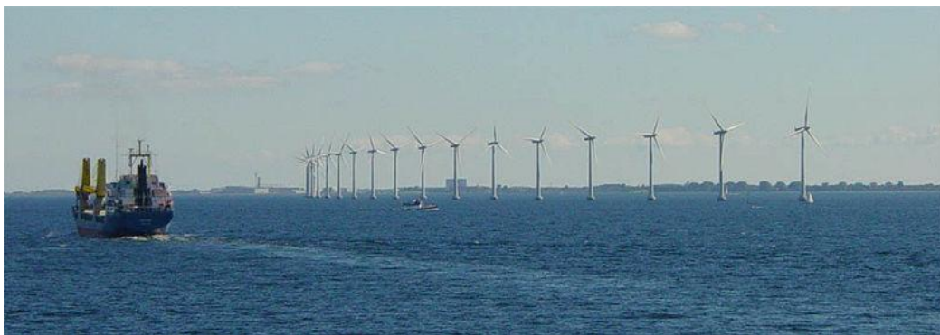
Modern offshore wind turbines near Copenhagen, Denmark.
