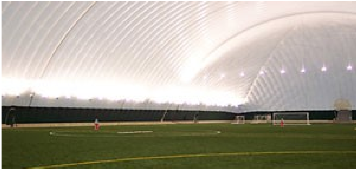
Inside of inflatable structure. New technologies allowed the Generations Sports Complex to cover an area 2 football fields in length by almost a football field wide without support columns to get in the way
