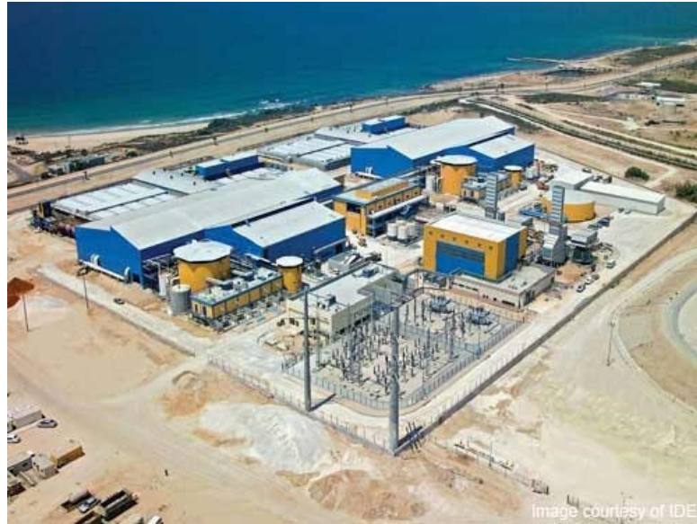
FIG.2A. ASHKELON SEAWATER REVERSE OSMOSIS (SWRO) DESALINATION PLANT, ISRAEL. PRODUCTIVITY 50M M 3 /YEAR (2006). COST USD $250M. (PICTURE HAS 34K).
