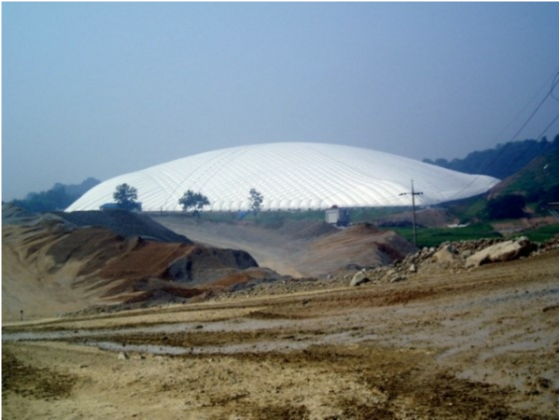
Current air support structures
