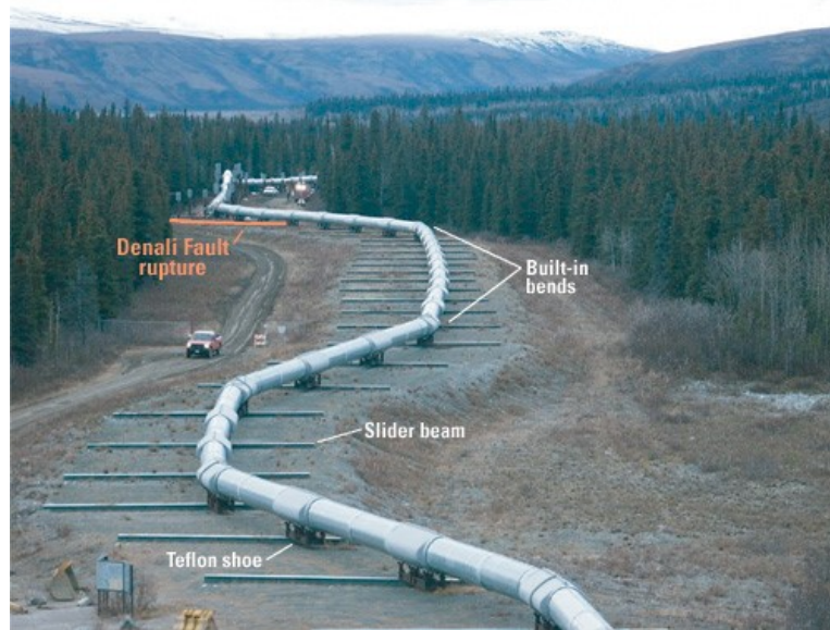
Trans-Alaska oil pipeline. Notice the damage.
