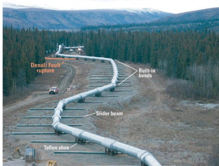
Trans-Alaska oil pipeline. Notice the damage.
