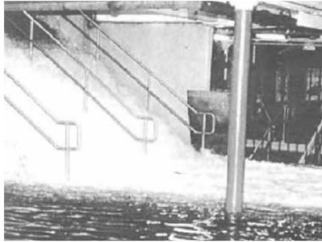
FIGURE 4-10C Hoboken PATH Station, New Jersey. 1992 Nor'easter.
