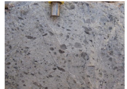
30D : Further Detail from site No : 30
