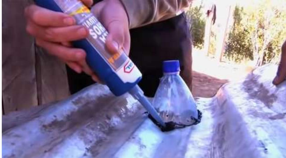
Figure 5. Installation process of Moser lamp (8)
